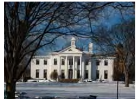
Front Exterior View
