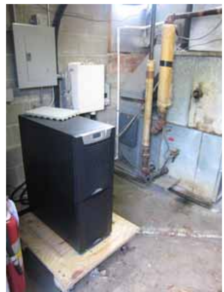
UPS Battery Backup
