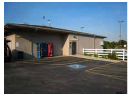
View of Entry
