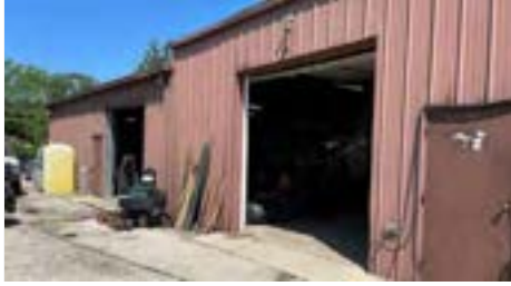
Sugar Creek Maintenance Building 2017 Score: D 2023 Score: Poor
