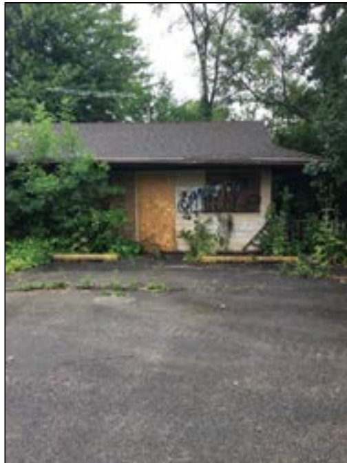
2 - View of the subject site abandoned office structure
