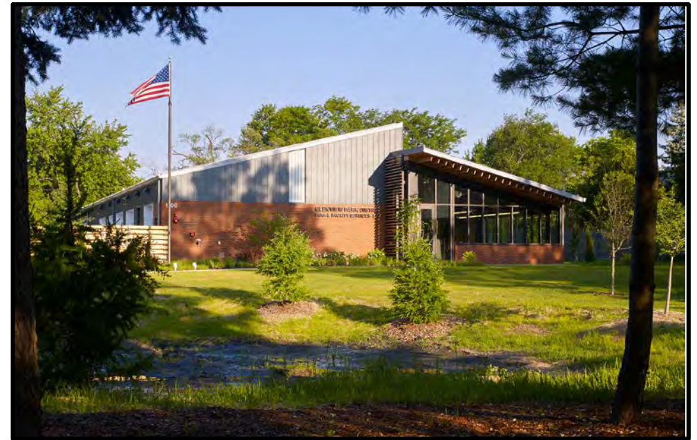
Glenview Park District's New Maintenance Facility
