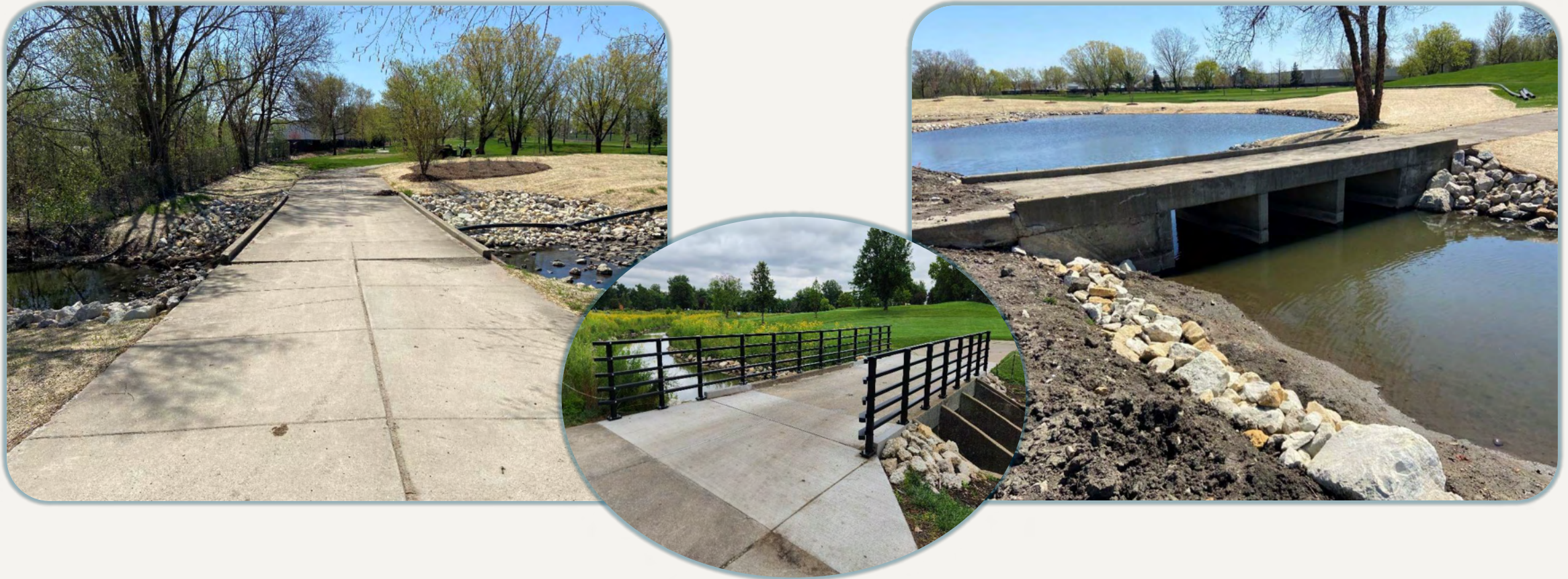
East and Central Bridge Repairs and Improvements $162,000
