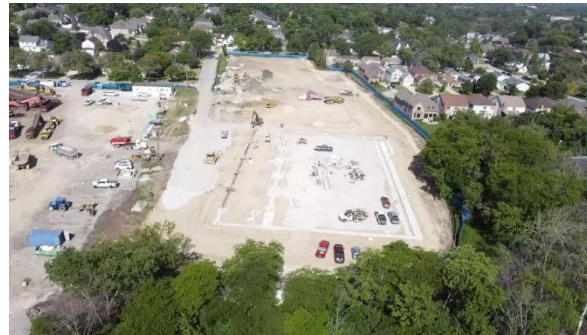
New Wagner Community Center Construction
